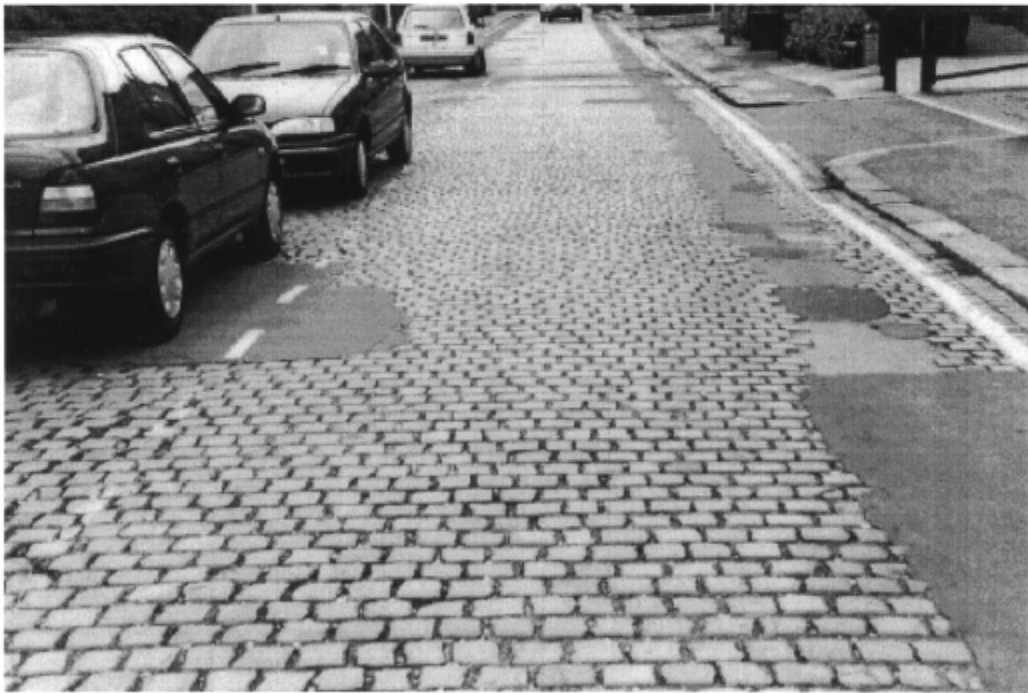
Figure 1. Two road surfaces used in the current study (a) Speedbump (Rampton Road) (b) Pave' (Mary Street).
